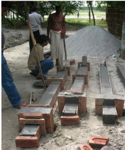
Figure 10: Pre-cast pile foundations
